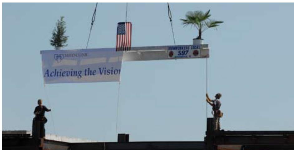
Workers place final beam of new hospital at Mayo Clinic Jacksonville.
